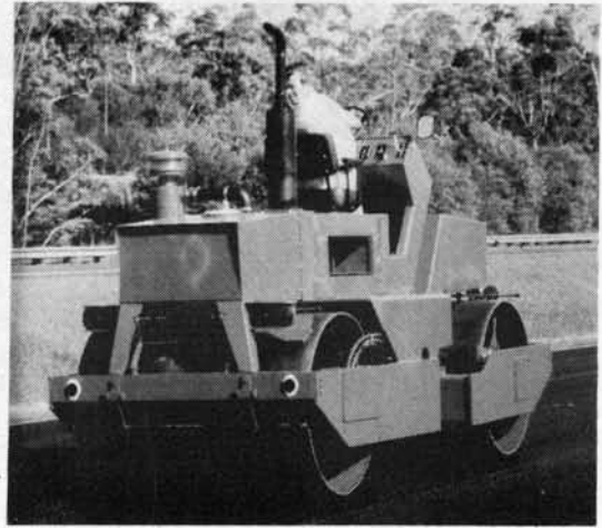
Pannell Plant 6 tonne Duplex DD1500 Double Drum Vibrating Roller working on the Newcastle Expressway at Mount White.
