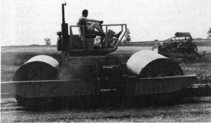
Pannell Plant 15 tonne Duplex DD2100 Double Drum Vibrating Roller working on the Southern Freeway.
